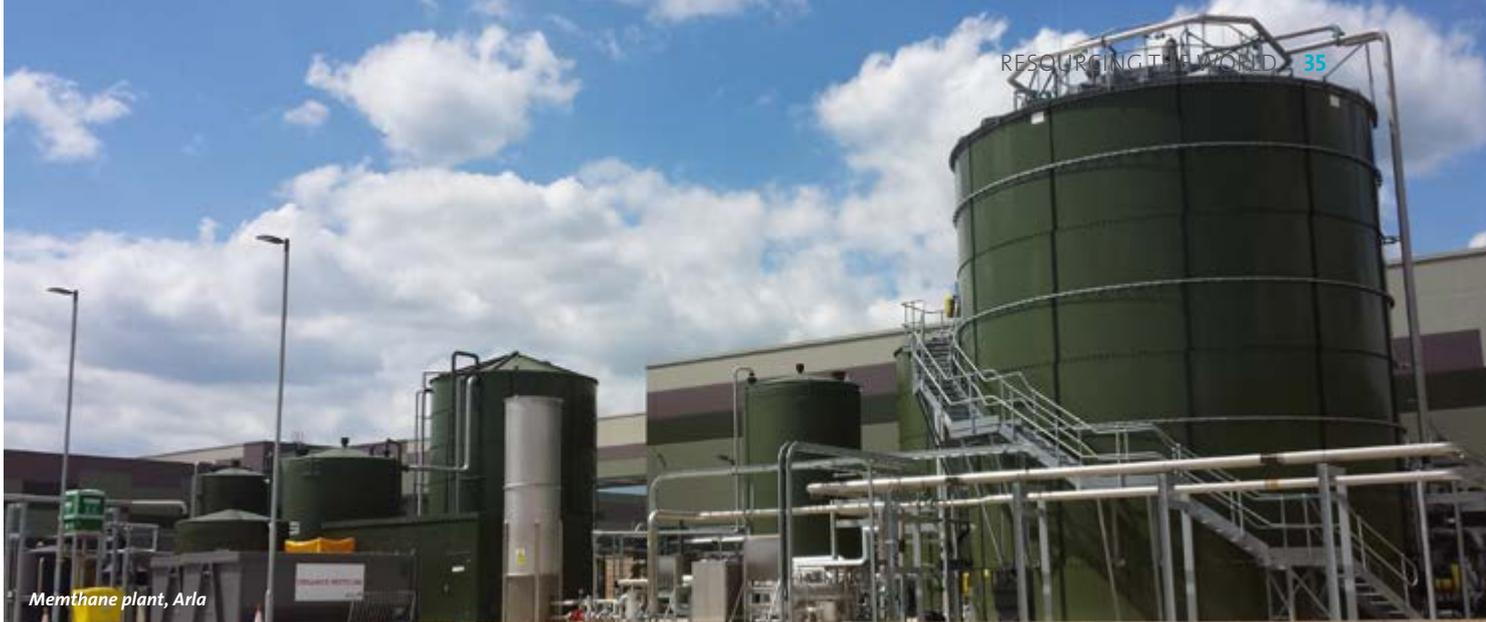
Advanced settlers are installed, which separate the biomass from the final effluent and the biogas. The system is designed for 2,800 m<sup>3</sup>/day of wastewater and produces more than 9,000 Nm<sup>3</sup>biogas per day (approx 2.8 MW).
