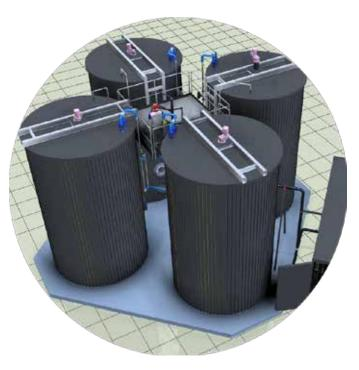
In addition to being the first Biofarm this ANITA<sup>™</sup> Mox plant was designed to treat up to 200 kg NH4-N/d with 85% total nitrogen removal and 95% ammonia removal.
